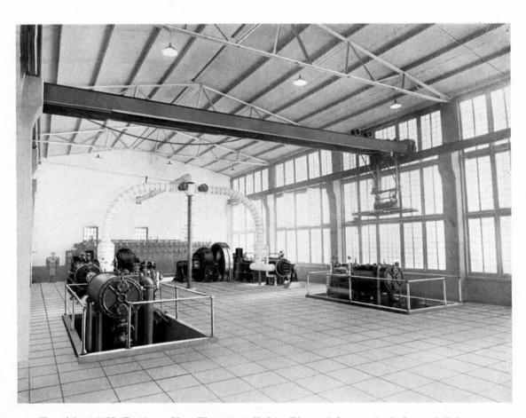
Two (2) 500 H. P. Ames Una-Flows installed in Plant of Compania Industrial Jabonera, Gomez Palacio Durango, Mexico. This entire design and installation including Engines, Generators, Switchboard, Condensers, and Superheaters, made by Ames Iron Works
